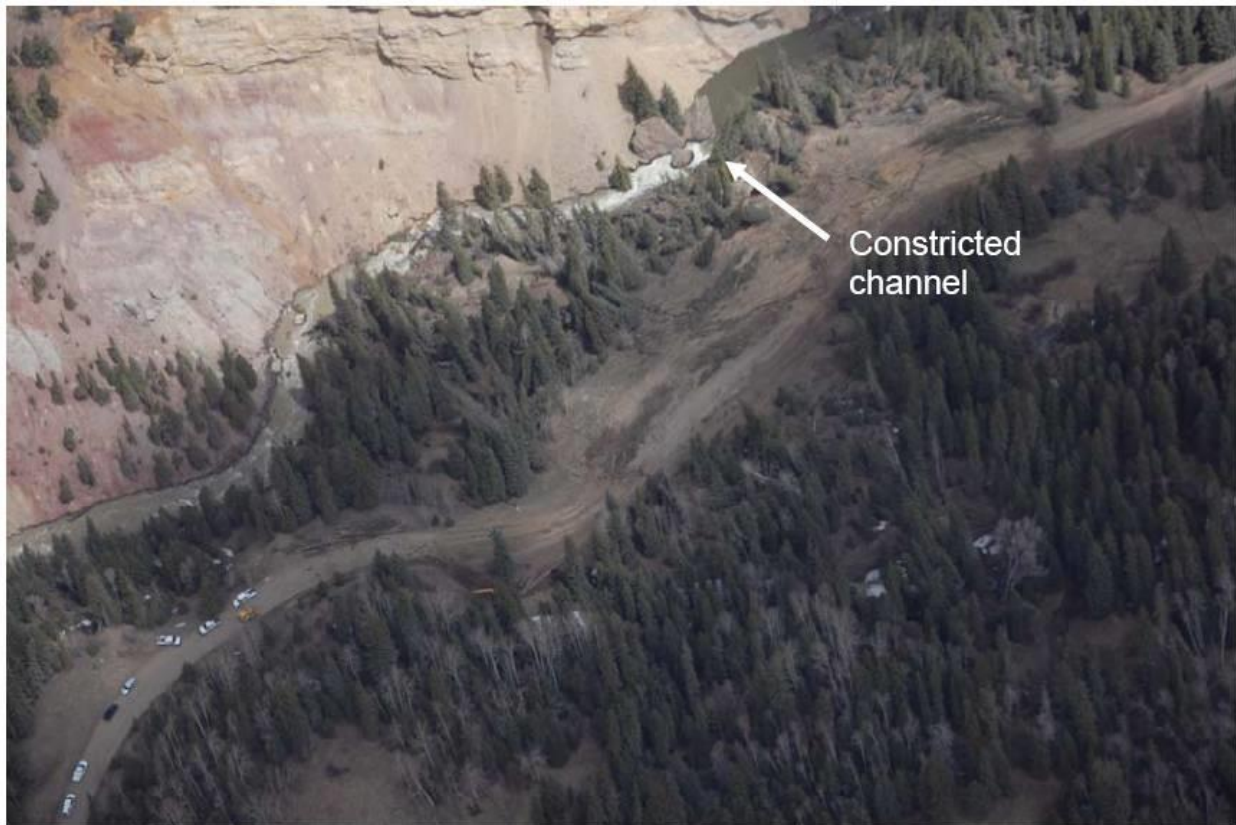
Figure 4 .24. Con str iction of the San Ju an River by the Toe of the Eas t Fork Land slide
