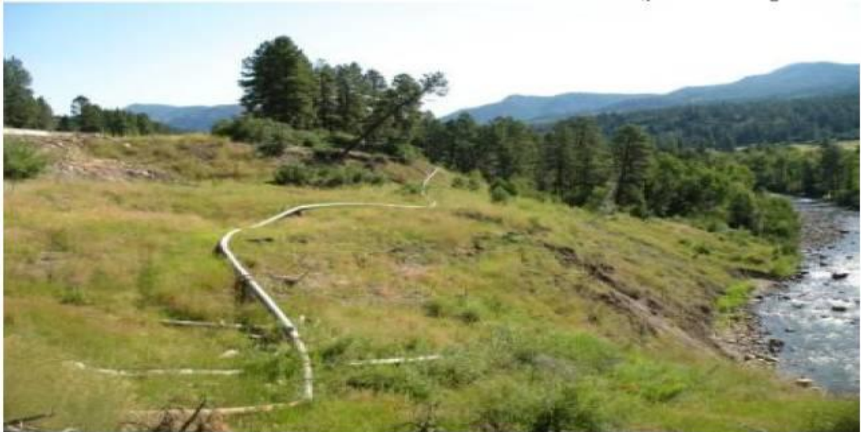
Source: MWH Americas, Inc., Final Report for the Snowball Pipeline Replacement Evaluation in the Vicinity of U.S. Highway 160 Jackson Mountain Landslide
