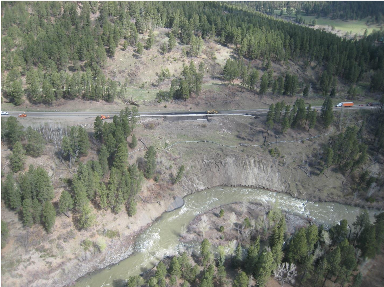
Figure 4 .22. Jackson Mountain Landslide Aerial View
